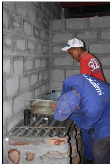
Making the basin base
